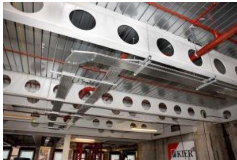
Figure 1: Structural cold-formed steel sections with perforated web.
